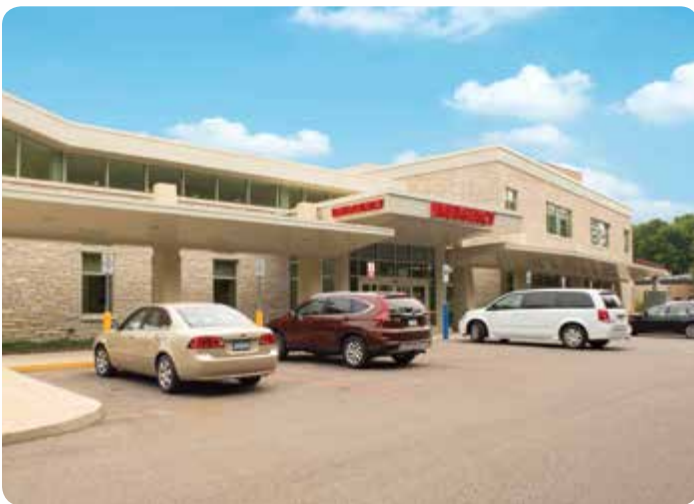
Recently renovated emergency entrance at St. Joe's Chelsea
